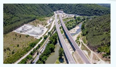
**Do you know that:** "Zheleznitza" tunnel is the longest and most modern road tunnel built so far in the country. Its two pipes are about 2 km long each. The facility has four pedestrian crossings and another two for cars between the tubes, in case of an emergency for the passing and evacuation of people. 26 SOS combined niches have been built and an intelligent traffic management system has been implemented.
